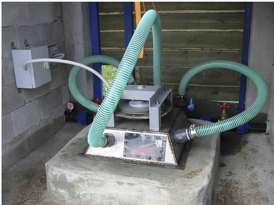
Fig. 4. A 500 W locally manufactured pico-hydroelectric plant.
