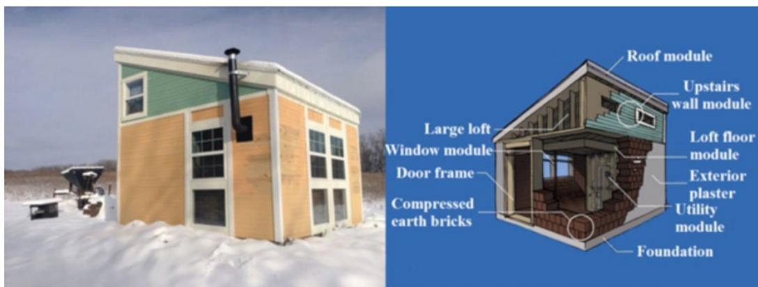
Figure 2: The OSE Microhouse project and its building modules Source: Adapted from Open Source Ecology, 2018
